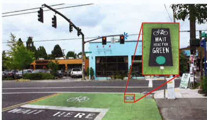
Figure 2: The 21st Avenue site Northbound approach with an inset image of the Modified Columbia Experiment Marking.
