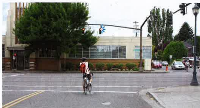
Figure 1: The Tillamook Street site Westbound approach.
